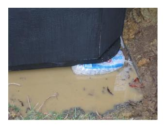
Figure 8. Swim Spa and Exercise Pool Position in Excavation on Ice Bag Allow the ice to melt and then the excavation will be ready for back fill with gravel.
