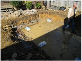
Figure 7. Ice Bag Positioning in Excavation
